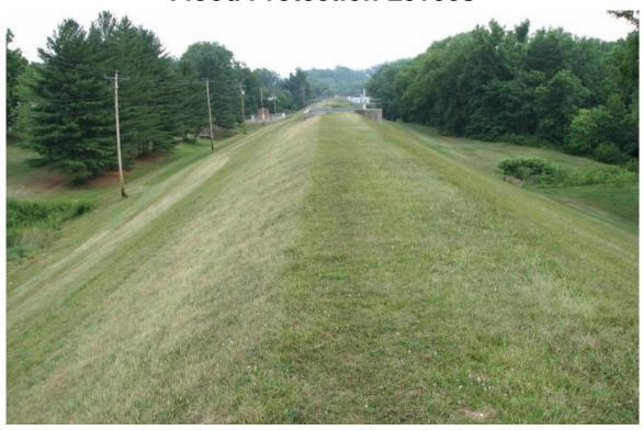
When rains are heavy, a 26-foot-high, 19,536-foot-long levee and floodgate system protects downtown Barbourville in Knox County from Cumberland River flooding. Photo by Dan Carey, Kentucky Geological Survey.
